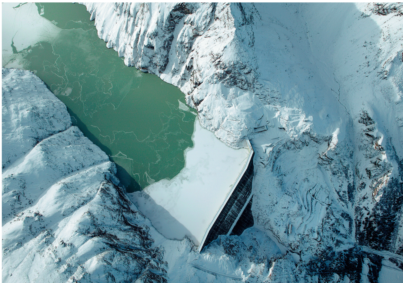
Staumauer Grande Dixence.
